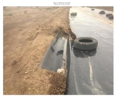
On both sides of each run dig a drench (approx. 250mm deep by 350mm wide) to lay the plastic edge into and then backfill to ensure the edges are secured. If using silo/light plastic, place tyres in the centre of the V to hold the plastic down.
